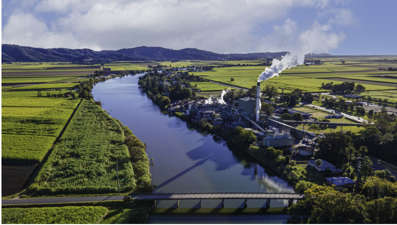
CondongSugarRefinery Merit Stefan Botczek
